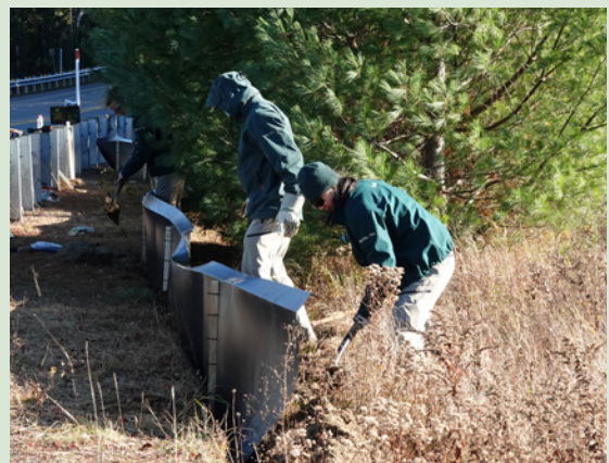
Employees doing maintenance work
