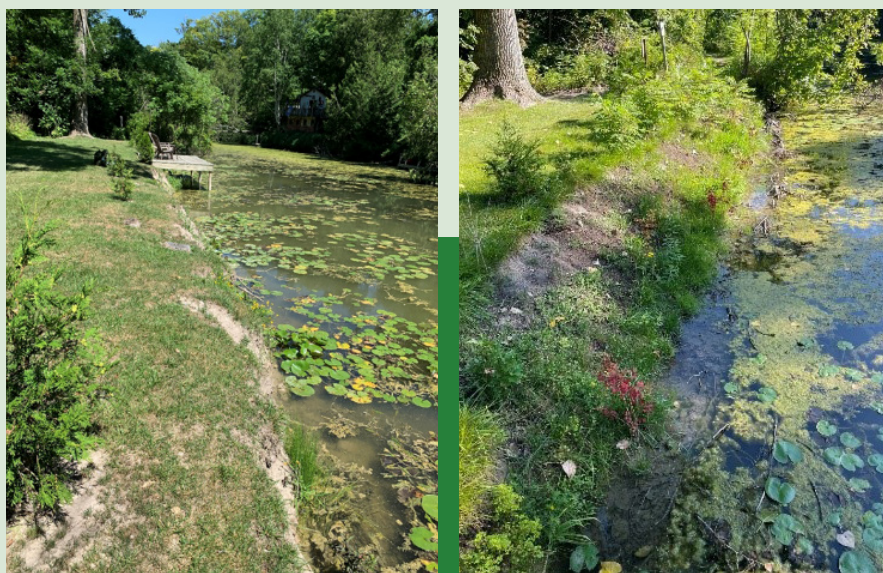
Photo to the left: Old Ausable Channel before bank restoration. The photo on the right is the same site where visible benefits are perceived after restoration – reduced erosion, reduced runoff, sediment accumulation allowing habitat for native species.
